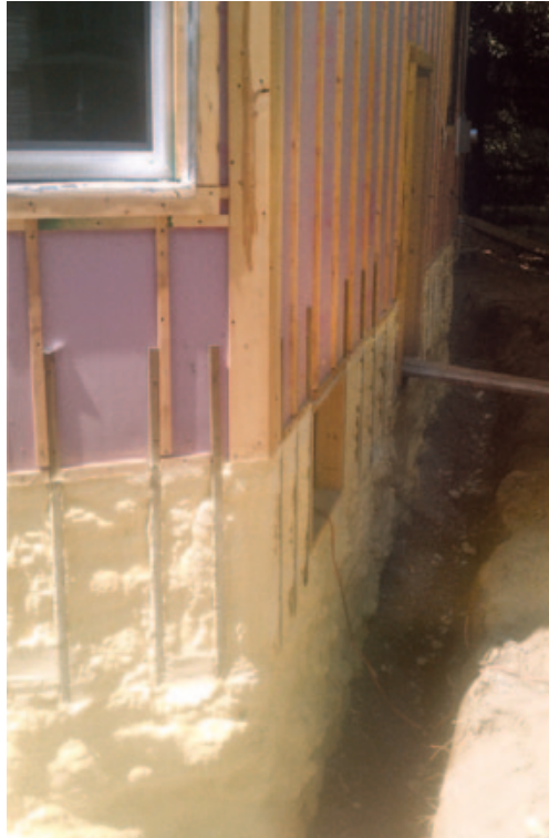
Most foundations in the DER houses needed waterproofing anyway, creating an opportunity to add foam to all of the foundation exteriors. Most received a double layer of rigid foam (far left); in two cases, spray foam — which served as a drainage plane — was the better choice (left).
