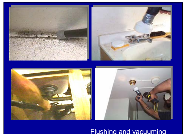
Flushing and vacuuming
